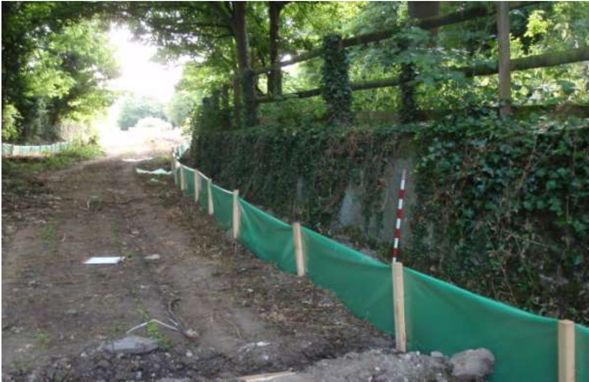
Plate 5. Site defined by green reptile barrier, note concrete retaining wall (looking east)
