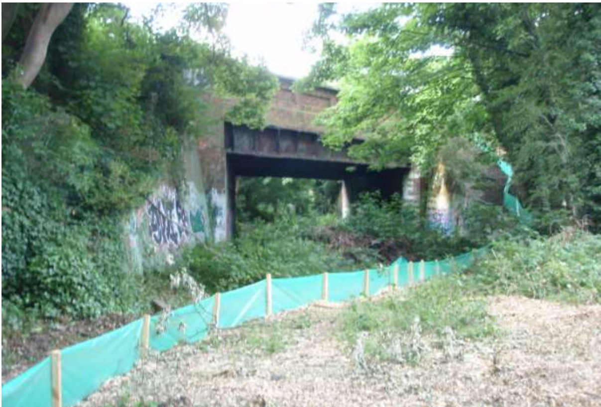
Plate 6. Railway bridge (outside the PDA and looking south-west)
