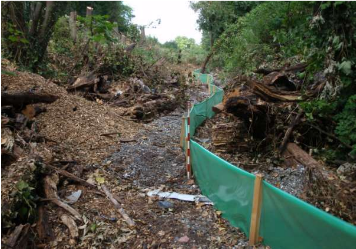
Plate 9. Further on- note roadstone of relict railway track (looking west)
